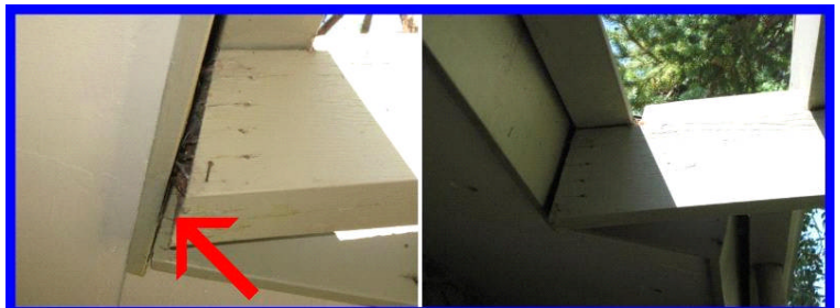
Inadequate support at patio
