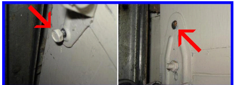
Loose or missing hardware
